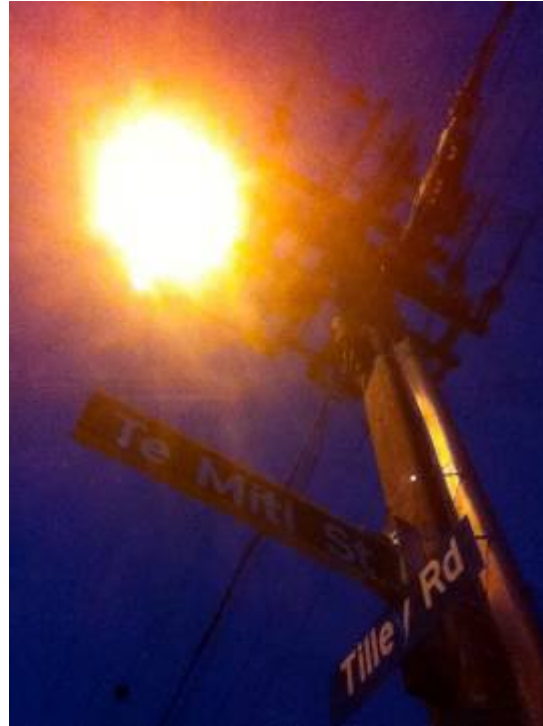
High Pressure Sodium - 89 Watts - life of 4-5 years
