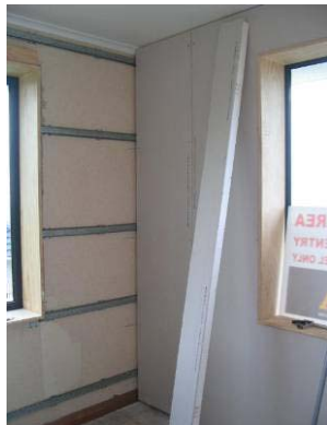
Figure 11. Wall insulation system: Expanded Polystyrene with Gib.
