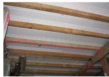
Figure 16. New underfloor insulation: Expanded polystyrene sheets.
