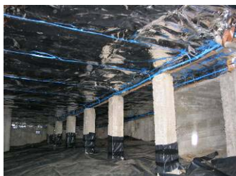
Figure 15. Existing underfloor insulation: Aluminium foil.
