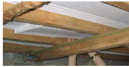
Figure 29. EPS panels under the floor.
