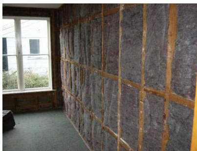
Figure 17. Wool batts placed inside of the existing walls.
