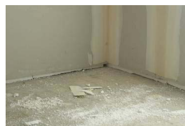
Figure 28. Fitting wall insulation (Formaliner)
