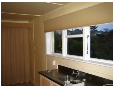
Figure 13. Existing single glazed wooden frame windows
