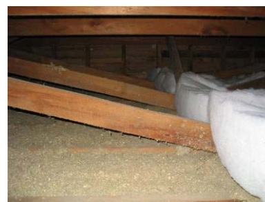
Figure 22. Ceiling insulation: Polyester blankets installed on top of existing macerated paper
