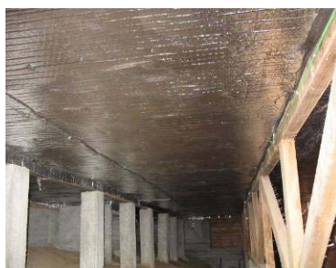
Figure 21. Underfloor insulation: Air-Cell
