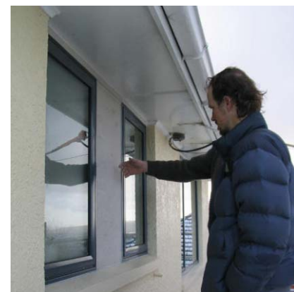
Figure 24. New Aluminium framed windows
