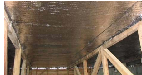
Figure 30. Air cell under floor insulation.
