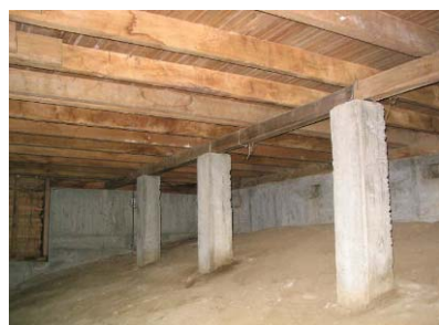
Figure 20. Floor non insulated
