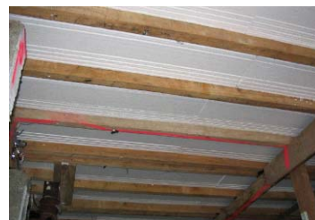
Figure 16. New underfloor insulation: Expanded polystyrene sheets.
