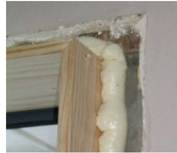
Figure 25. Foam around window seal in new windows
