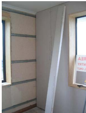
Figure 11. Wall insulation system: Expanded Polystyrene with Gib.
