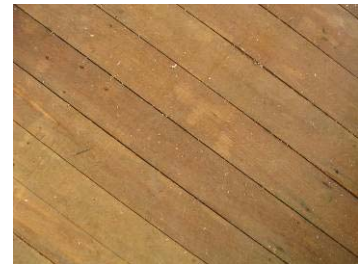
Figure 26. Wooden floor showing existing gaps
