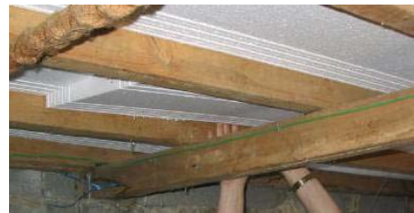
Figure 29. EPS panels under the floor.
